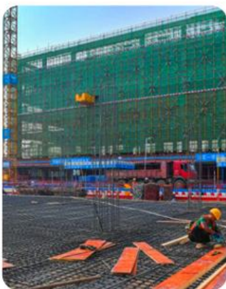
Construction Site Dust & Gravel Removal
